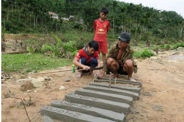
Figure 1 Villagers are making concrete landmarks
